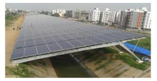
Fig. 4. The Canal-top Solar [6]
